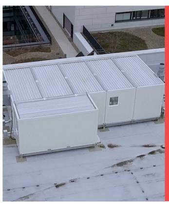
The project consists of 6 containers according to cleanroom class <6 according to DIN EN ISO 14644. 2 containers for HVAC system, HEPA filtration and technics. 4 containers for the use as cleanrooms. Components: Vertical laminar flow workbenches, PLC controlled hot plates, distilles, extraction unit for ultrapure water, weighing room, room for sample preparation and storage.
