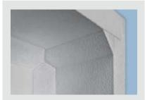
Gluing a triangular chamfer into the 90° corner creates an angled corner with a 45° angle.
