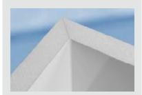
Joint compound is applied to the 90° corner and shaped into a chamfer.
